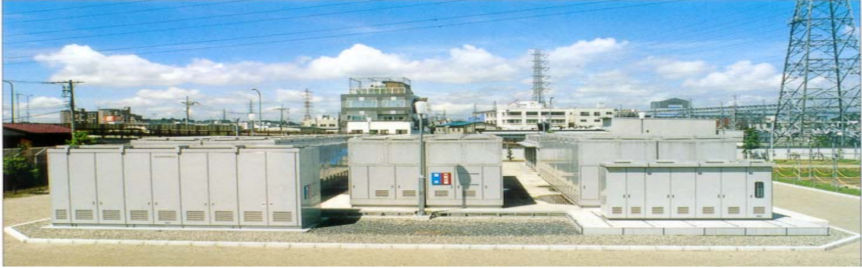
Fig. 9: Sodium sulphur high-temperature battery for load-levelling operation (Tokyo Electric Power Company, Tsunashima – 6 MW, 48 MWh).
